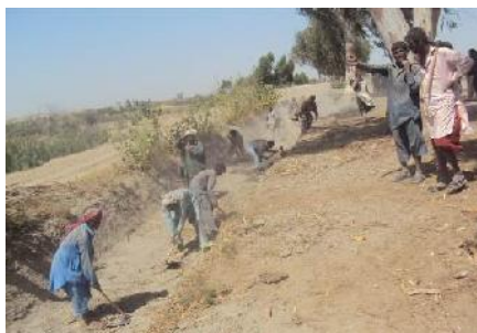
Figure 8- De-Silting under way
